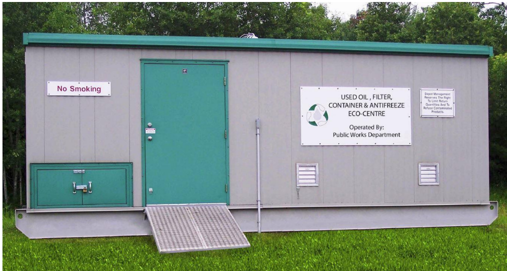
Eco-Centre with inside storage tank, secondary containment and storage for container bags, oil filter and antifreeze drums, equipment and supplies
