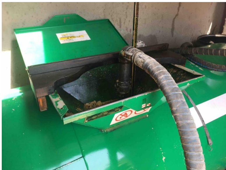
The Collector will hook a Hose to your Tank
