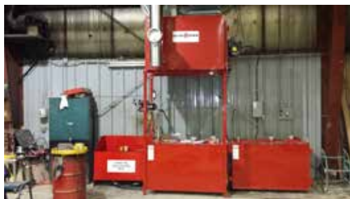
Used oil burner installed at the Public Works Garage
